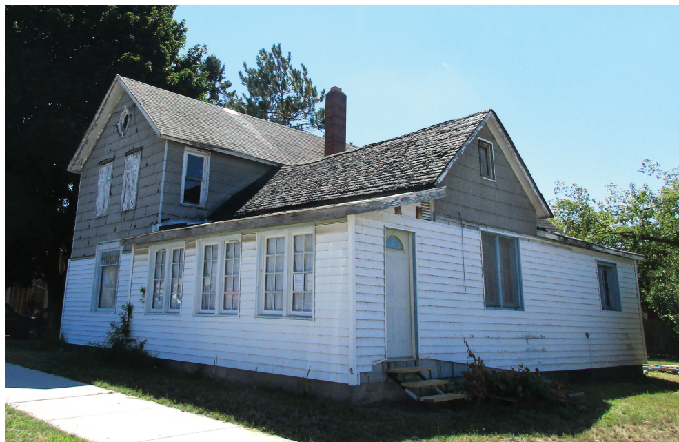
(PHOTO BY MICHELLE MEDJESKY) The Boyne City Commission has finally authorized the demolition of this vacant house at 204 S. East Street, where for years it has stood as an eyesore and matter for neighbors' concerns.
